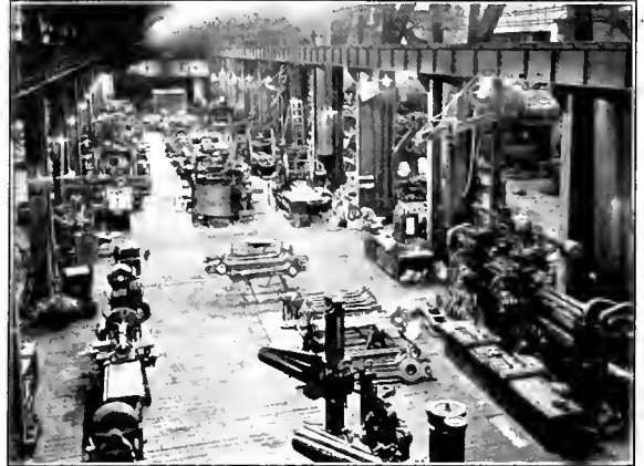
Fig. 3—Machine Shop Crane Bay Under Its Own Illumination—Note the Absence of Shadows
